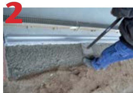
2 Pour concrete bed - 12" wide by 4" deep; keep outlet pipe clean.
