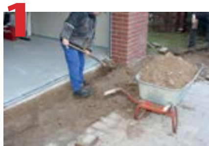
1 Excavate area to allow room for channels/catch basin and 4" of concrete on all 3 sides.
