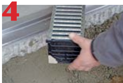
4 Fit end caps. Insert grates. To keep concrete from getting onto grates or seam, protect grates with plastic.
