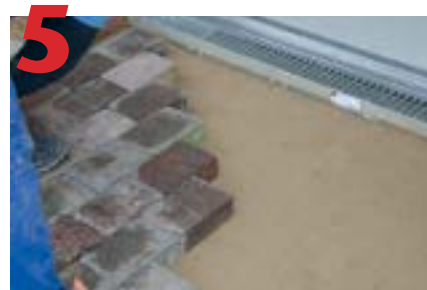
5 Install pavers or finish pavement surround to required level. Should be 1/8" above grate.
