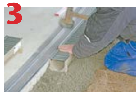
3 Lay channels starting at outlet. Set a string line at required height to ensure level. Seal joints if required.
