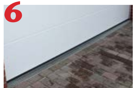
6 Clean away debris, remove protective plastic.
