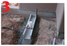
Lay channels starting at outlet. Set a string line at required height to ensure level.
