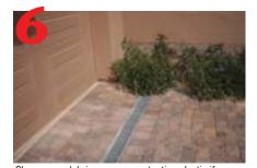
Clean away debris, remove protective plastic if necessary. Seal joints if required.
