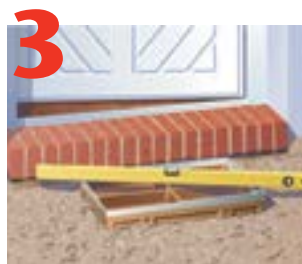
3 Level base unit. Backfill surround with concrete and finish surface as desired (tile, paver, etc.).
