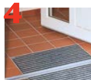
4 Install mat and installation is complete.
