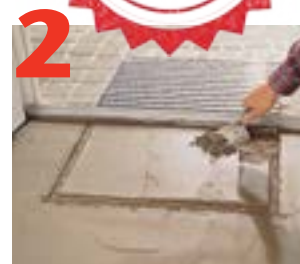
2 Excavate area large enough to fit DrainMat base.
