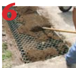
Fill voids in with gravel or soil. Use back of rake to spread evenly to top of GrassGrid.
