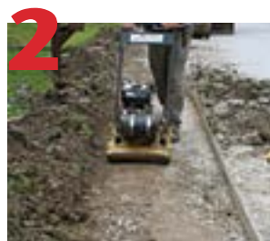
Spread fill/bedding layer evenly, compact well.
