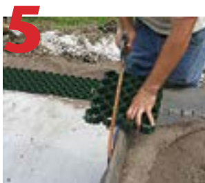
GrassGrid is easily cut using a hacksaw.
