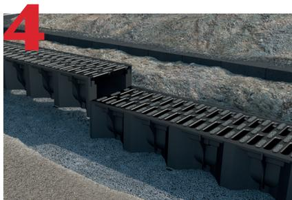
Continue to lay channels working away from outlet, channels slide-fit together.
