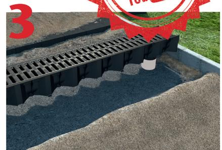
Knockout channel base for outlet and start to lay channels from outlet position.
