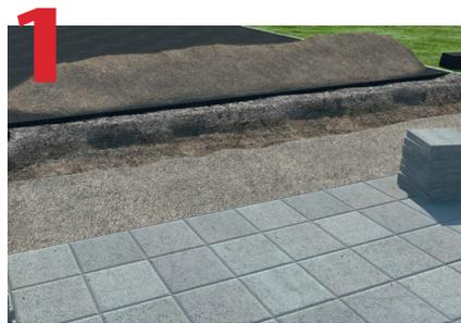
Excavate area to accommodate trench drain and 4" concrete surround.
