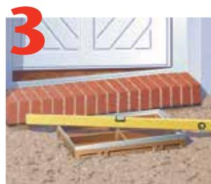
Level base unit. Backfill surround with concrete and finish surface as desired (tile, paver, etc.).
