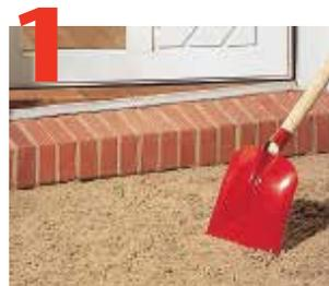
Excavate area large enough to fit DrainMat base, add 2" sand and compact well.
