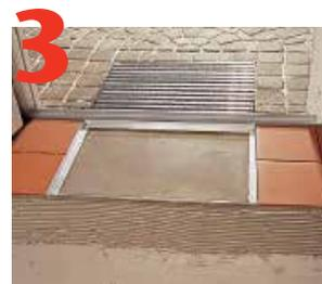
Install MatFrame, tile floor ensuring surface is 1/8" higher than MatFrame to prevent trip hazard.
